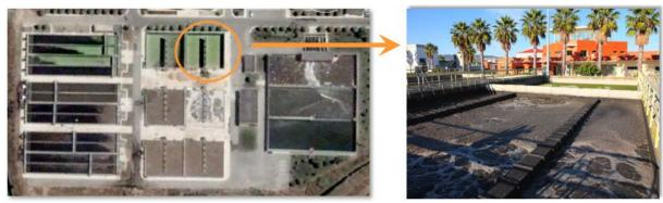
Figure 13. Conversion of reactor nº6 of Frielas WWTP to Nereda<sup>®</sup> technology.
