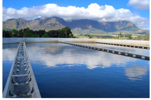
Figure 10. Nereda<sup>®</sup> reactor at Wemmershoek discharging effluent.
